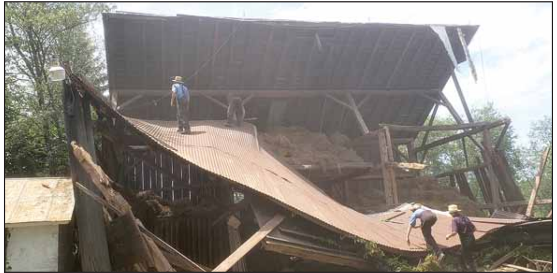
Workers from Mountain View Enterprises dismantle the nearly 200 year old barn on the historic Wech property in Wright Township earlier this month.
